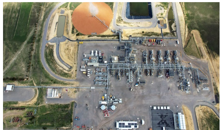
Image: Waitsia Gas Plant.
