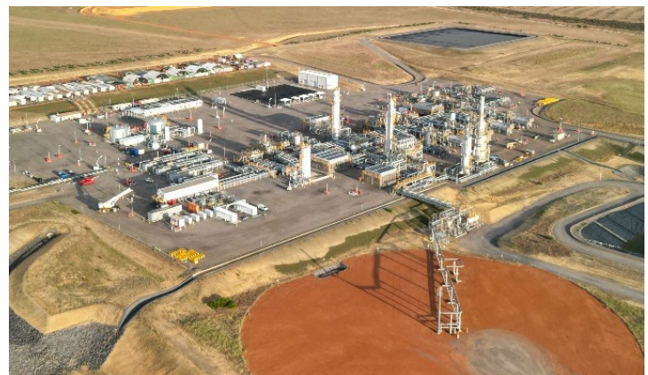
Image: Waitsia Gas Plant.
