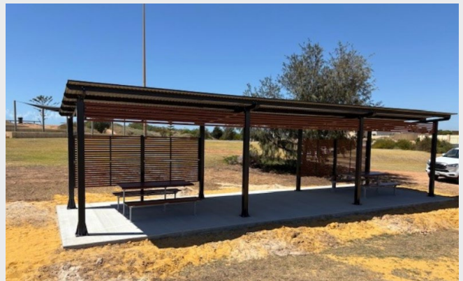
Image: New shelter installed at the Port Denison Skate Park Precinct.
