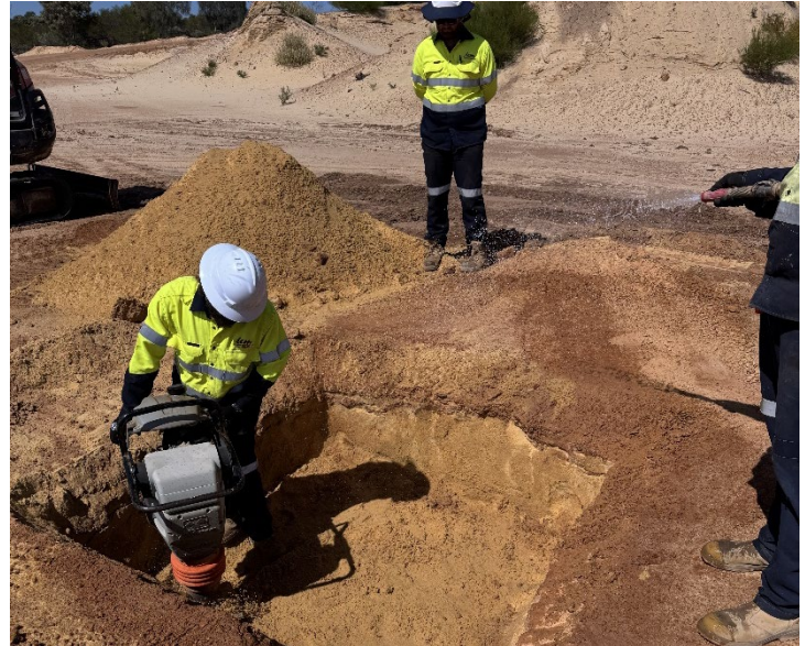
Image: ICM team conducting compaction testing at Waitsia-12.
