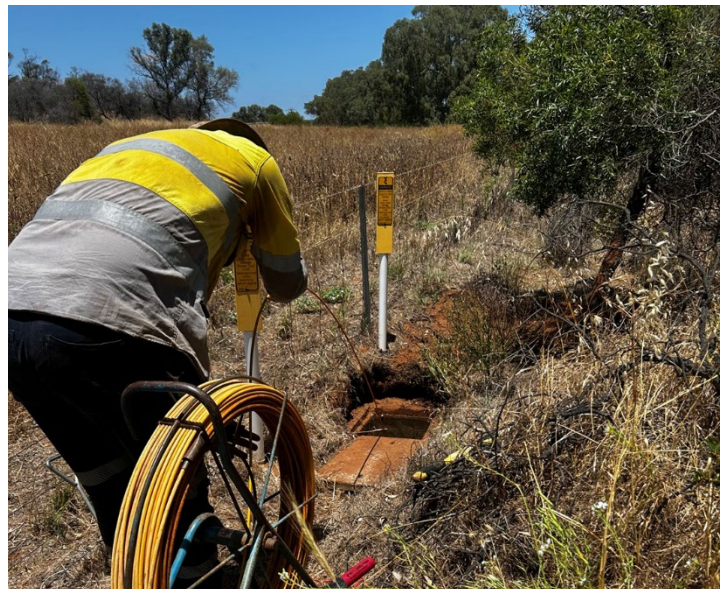
Image: Team locating Telstra fibre optic cable during potholing.
