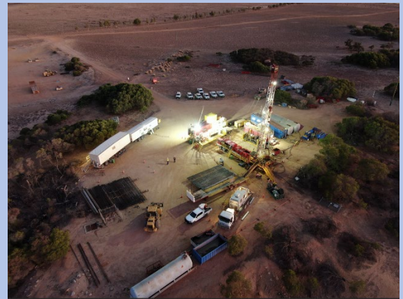
Image: Rig 226 conducting plug and abandonment operations at D21A in March 2024.
