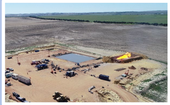
Image: Well testing at MEPAU's Waitsia-05 site.
